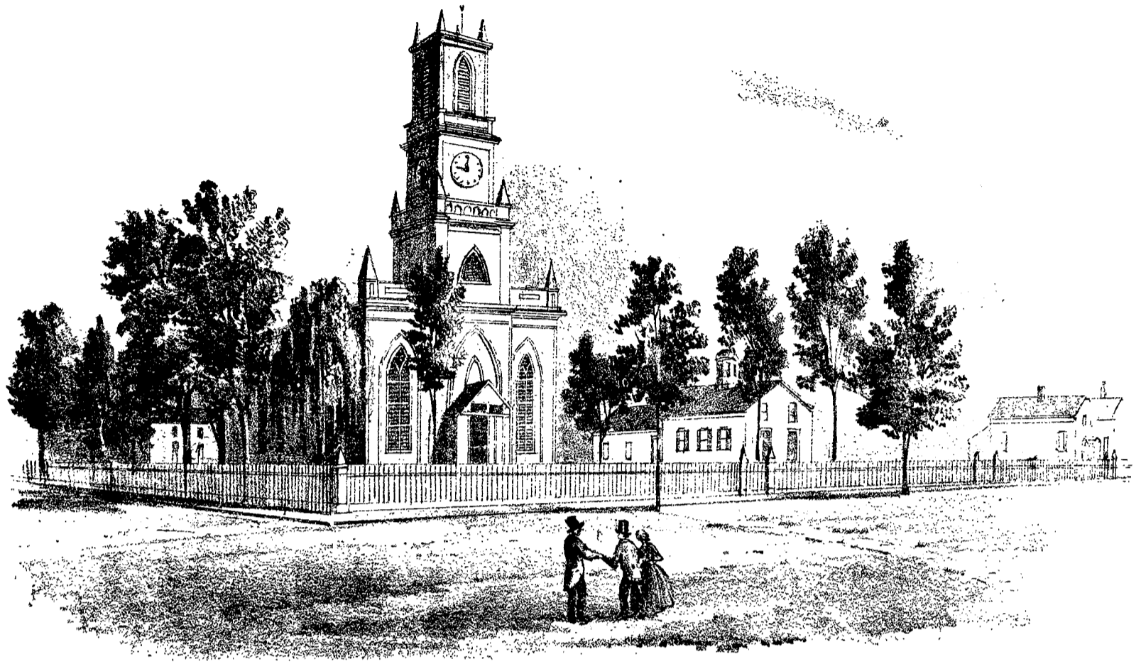
St. Paul's (Episcopal) Church & Parish School Waterloo
