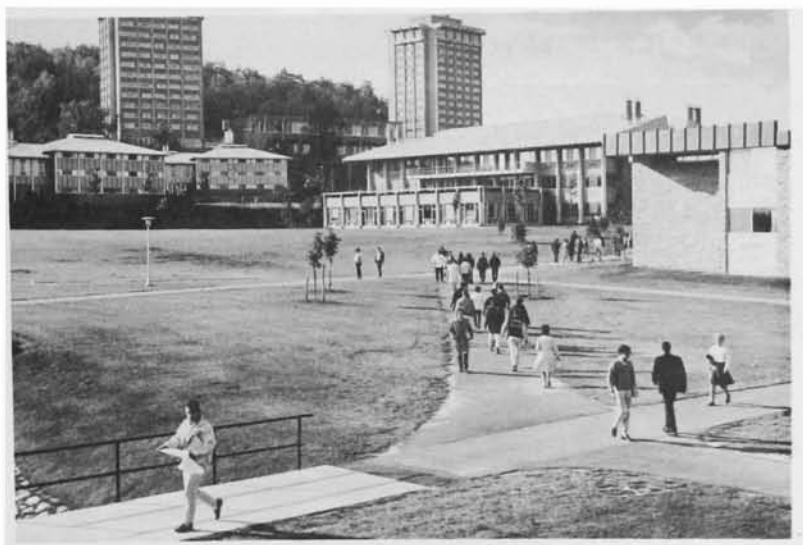
Part of the new South Hill Campus of Ithaca College.
