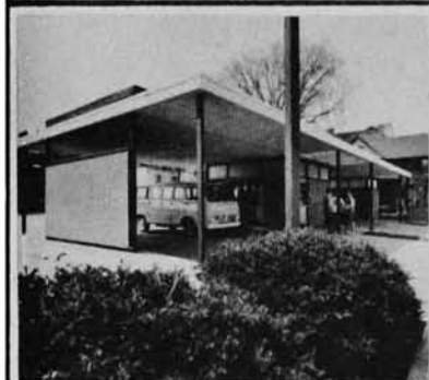
Drive-In Windows, E. Seneca St.
