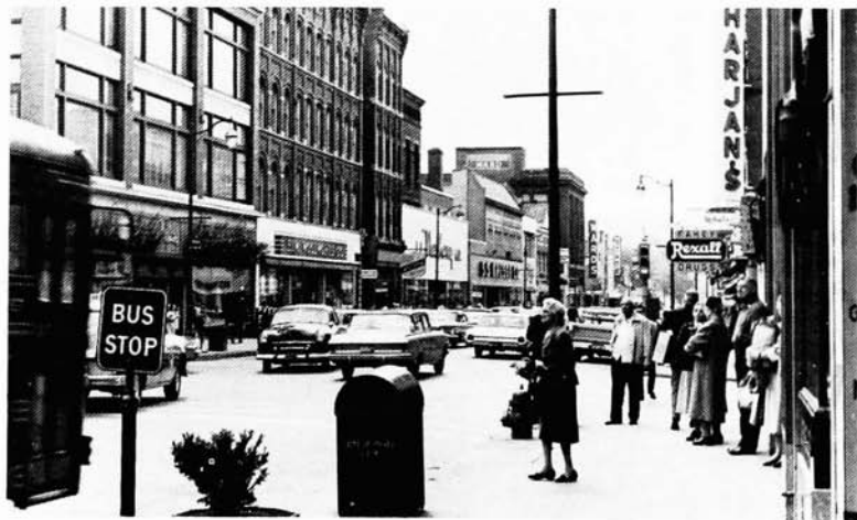
EAST STATE ST. LOOKING WEST
