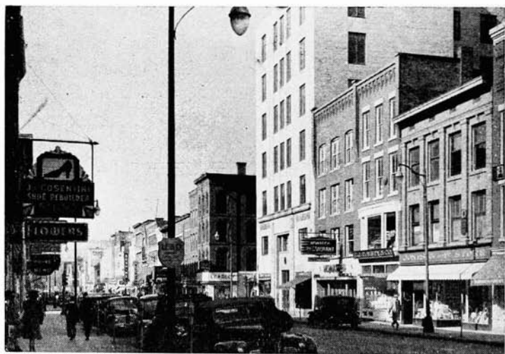
EAST STATE ST. LOOKING WEST
