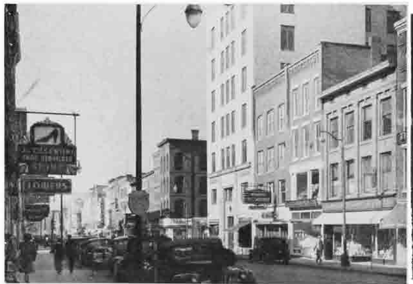
EAST STATE ST. LOOKING WEST
