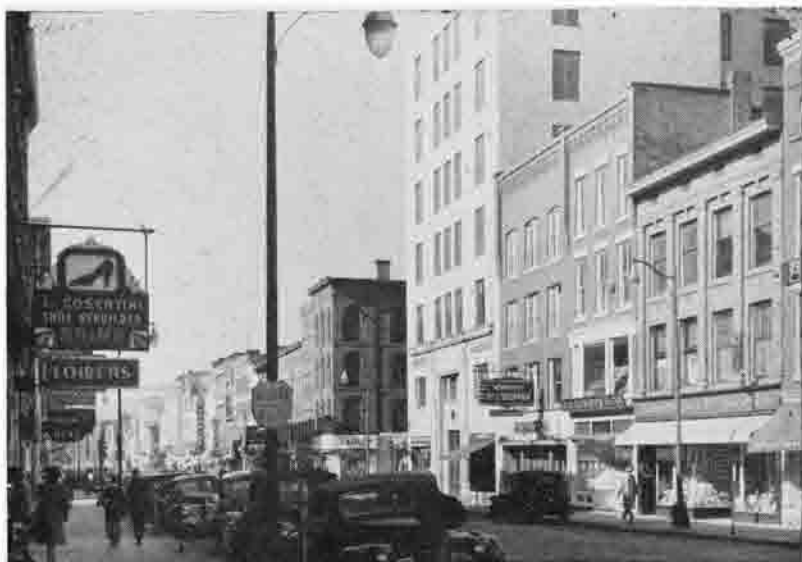
EAST STATE ST. LOOKING WEST
