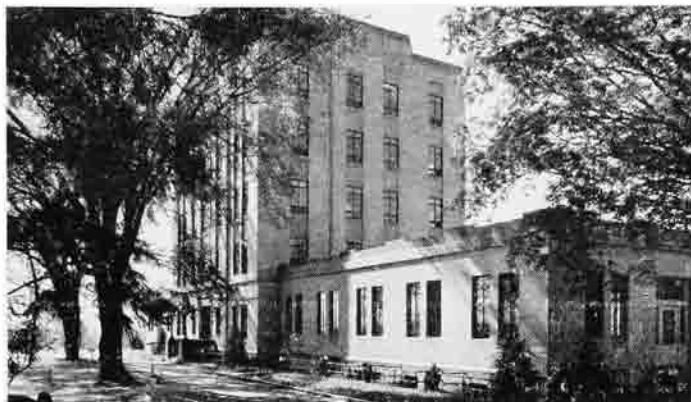
AN INDUSTRIAL BUILDING
