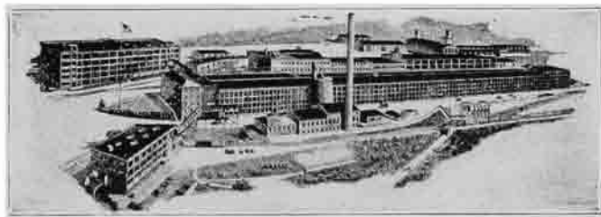
A MODERN INDUSTRIAL PLANT
