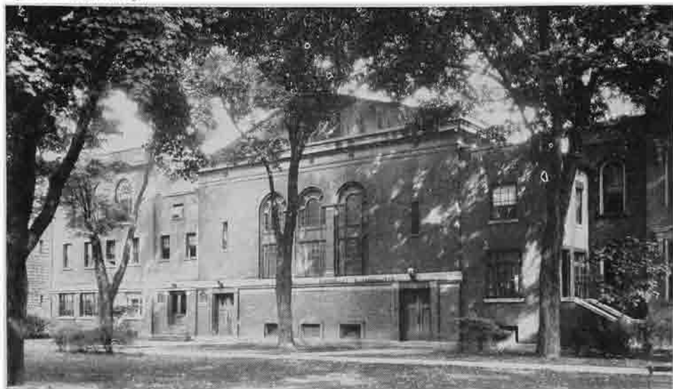
ADMINISTRATION BUILDING AND LITTLE THEATRE OF ITHACA COLLEGE
