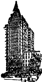
Company's Building 256 Broadway N. Y. City
