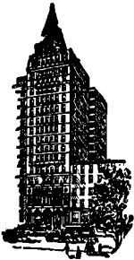
Company's Building 256 Broadway N. Y. City
