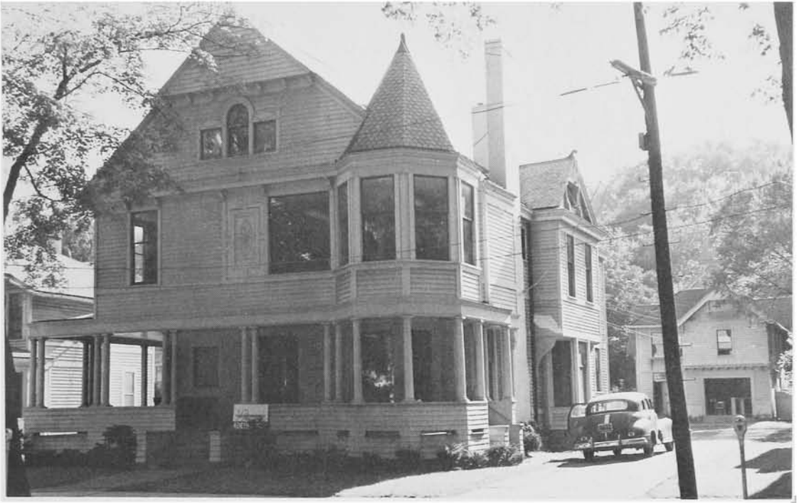
The Livermore Memorial Building, 313 North Aurora Street.
