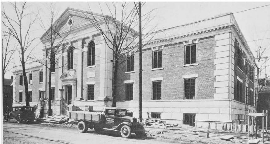
The Tompkins County Courthouse under construction.
