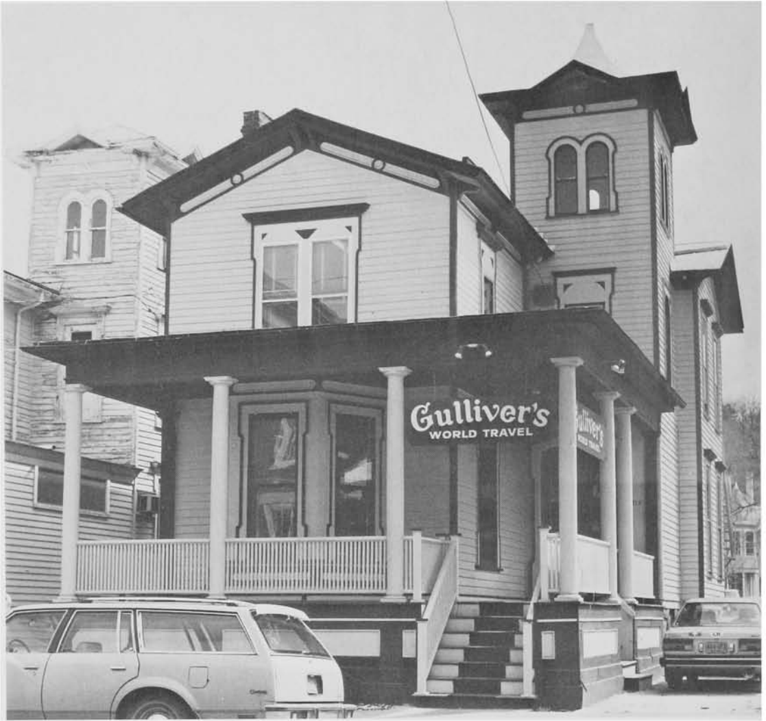
313 North Tioga Street. (Photograph by Carl Koski, 1981.)
