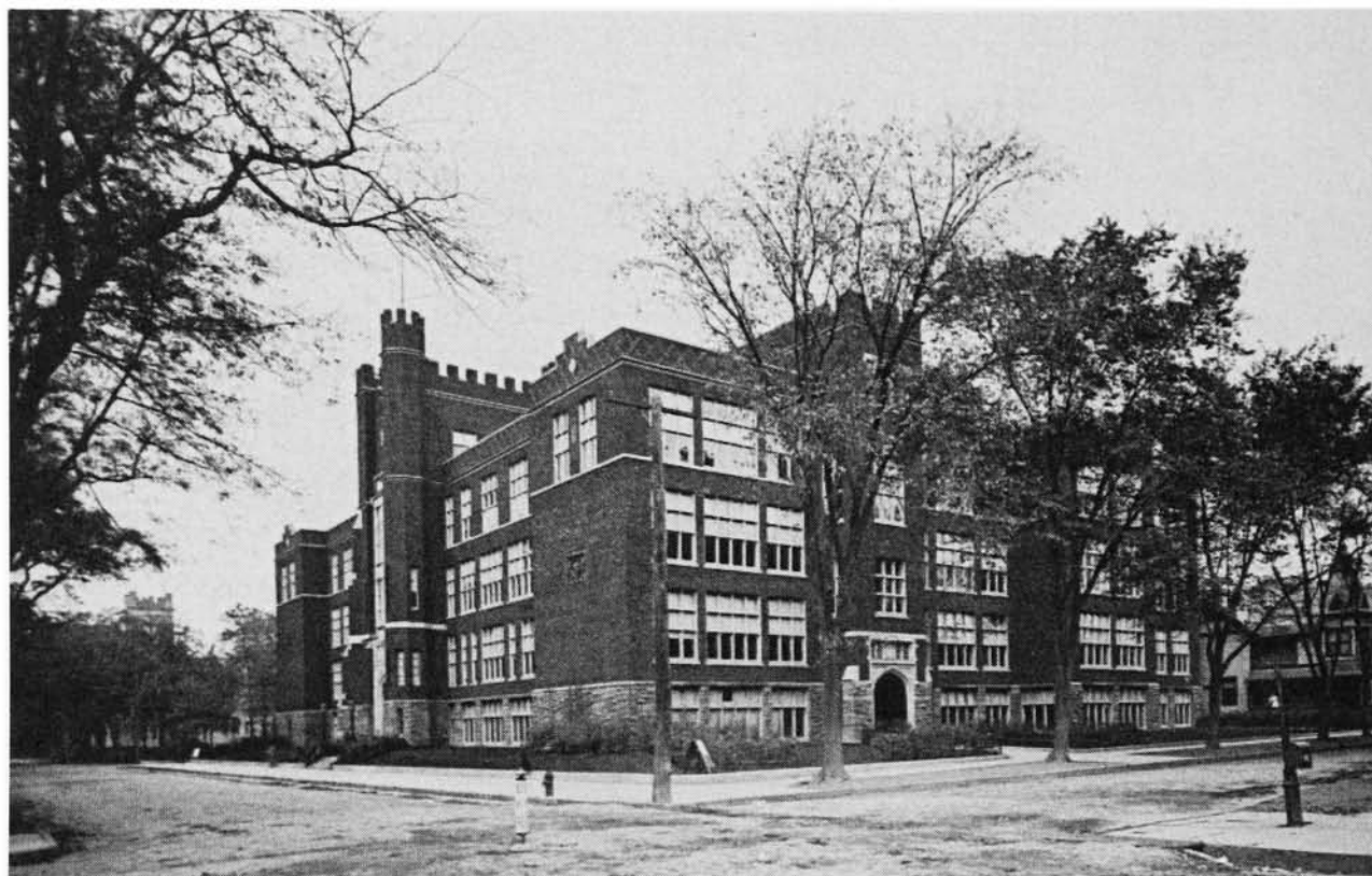
16. The DeWitt Building was designed by William Henry Miller in 1912 and housed Ithaca High School from 1912 to 1960 and DeWitt Junior High School until 1971. In that year it was sold to William S. Downing, Jr., who converted it to retail, office, and residential use.
