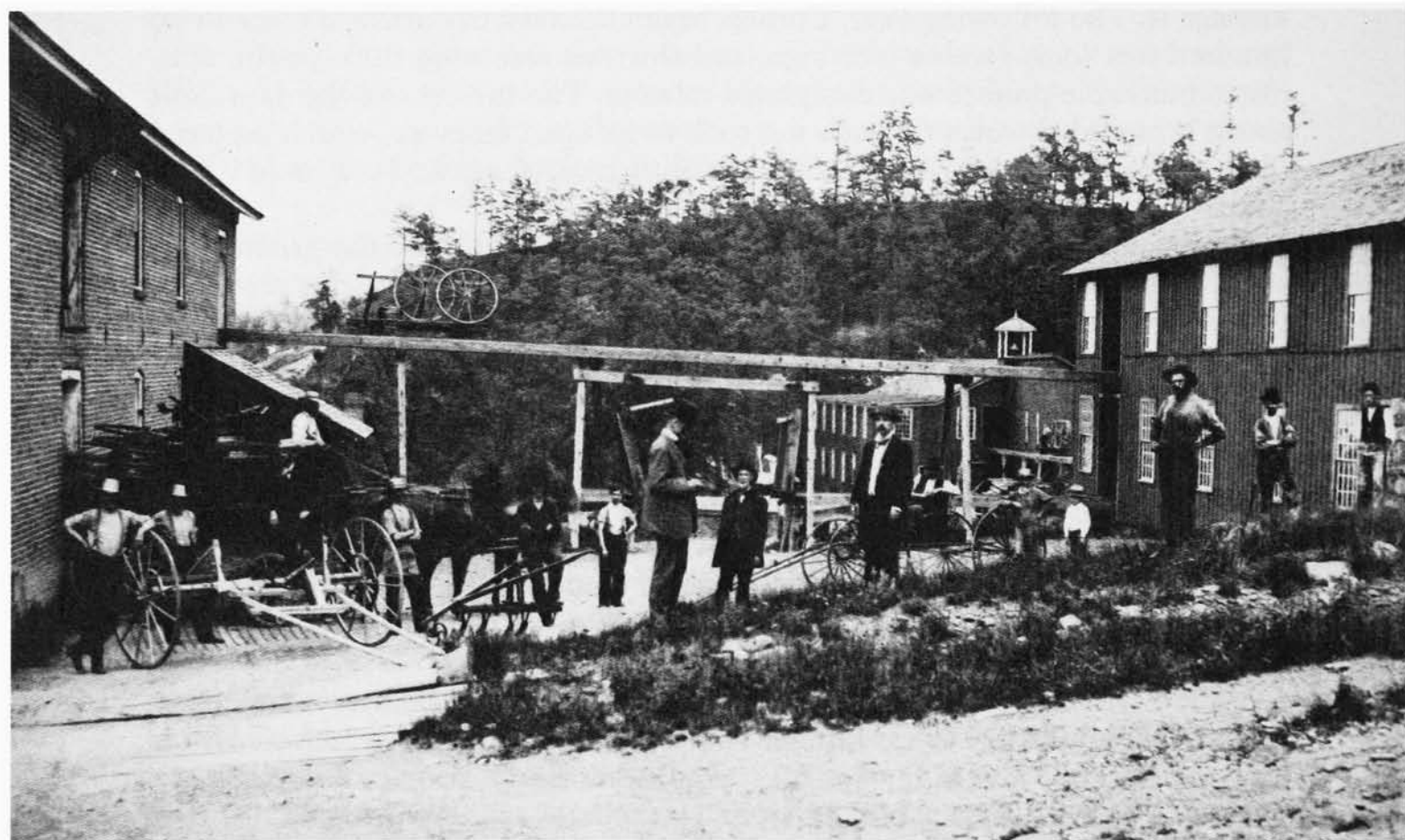
19. Two Fall Creek factories: (Above) The Ithaca Paper Company, ca. 1900. Paper was manufactured on this site almost continuously from 1819 to 1954. (Below) The Ithaca Manufacturing Works, ca. 1885. Rake parts were passed on an overhead ramp from the paint shop (right) to the storehouse (left).
