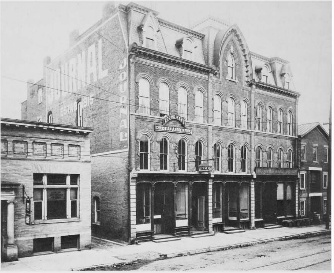
The Titus Block around 1905, before extensive renovation by the Ithaca Journal.
