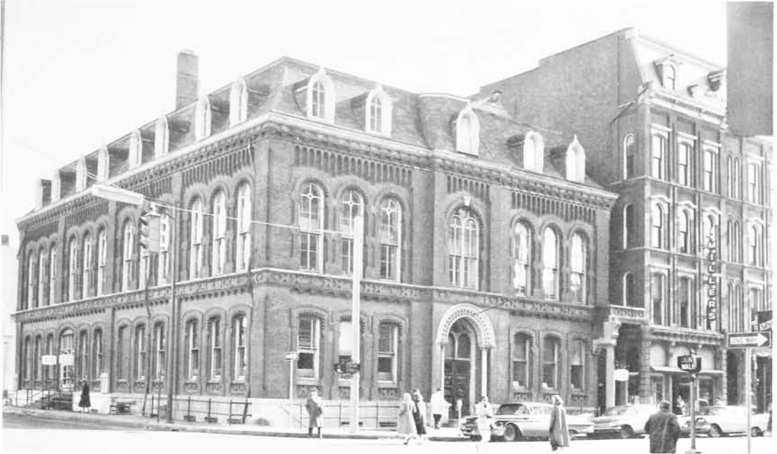
The Cornell Library, with part of the Blood Building on the right, around 1960 (since demolished). A handsome cupola on the library had been removed. (From the Henry Head Collection.)
