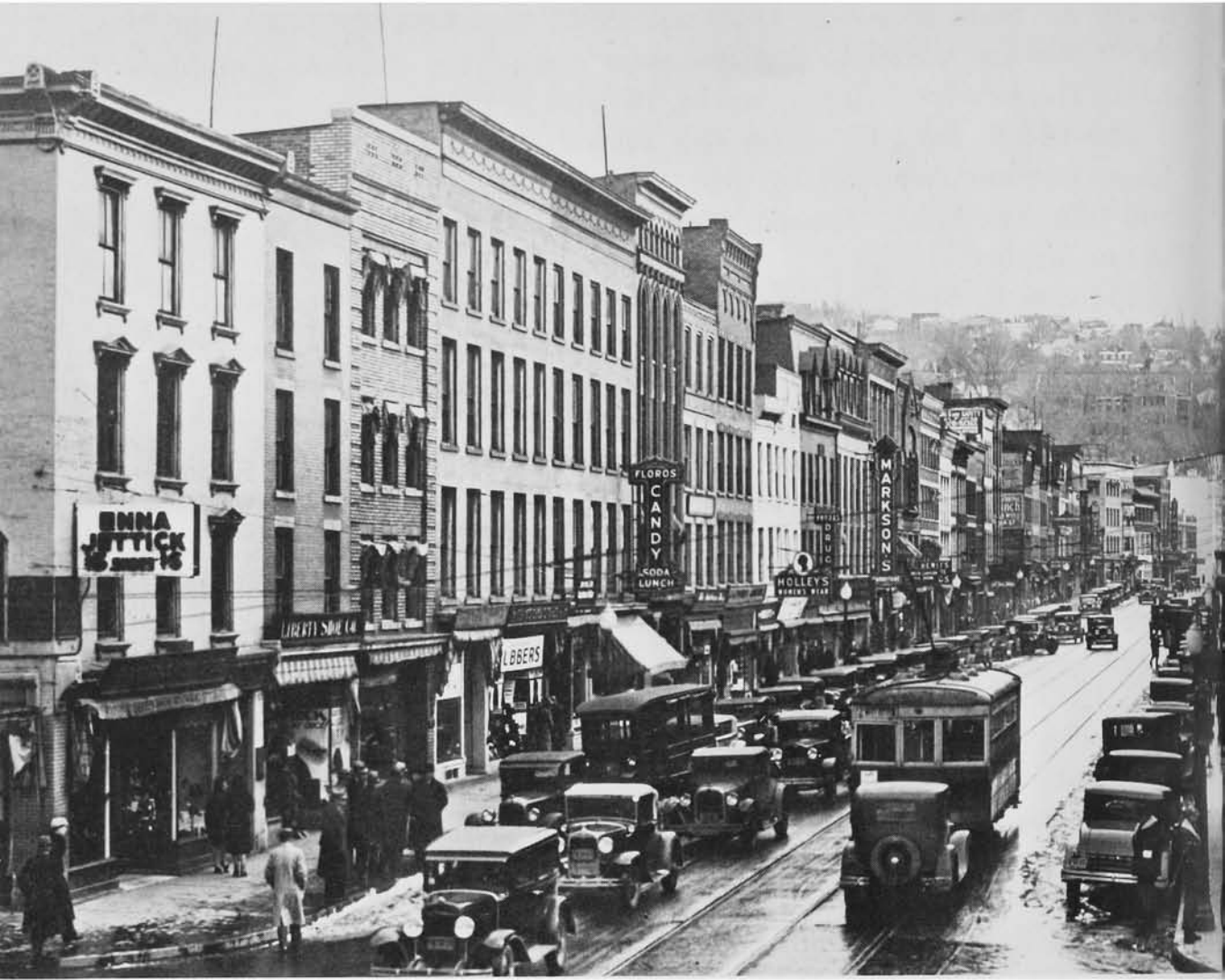
The 100 block of East State Street (north side), looking east from Cayuga, around 1930. On the left is the Baldini Building; three buildings to the right of it is the Grant Block. (From the Ralph Smith Collection.)
